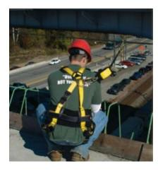
**Image 1.** A horizontal lifeline could prevent lanyards from making contact with exposed edges.
