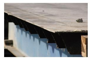
Image 2. Metal edges can cut lifelines and lanyards.
