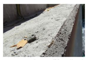
Image 3. Concrete edges can cut lifelines and lanyards.
