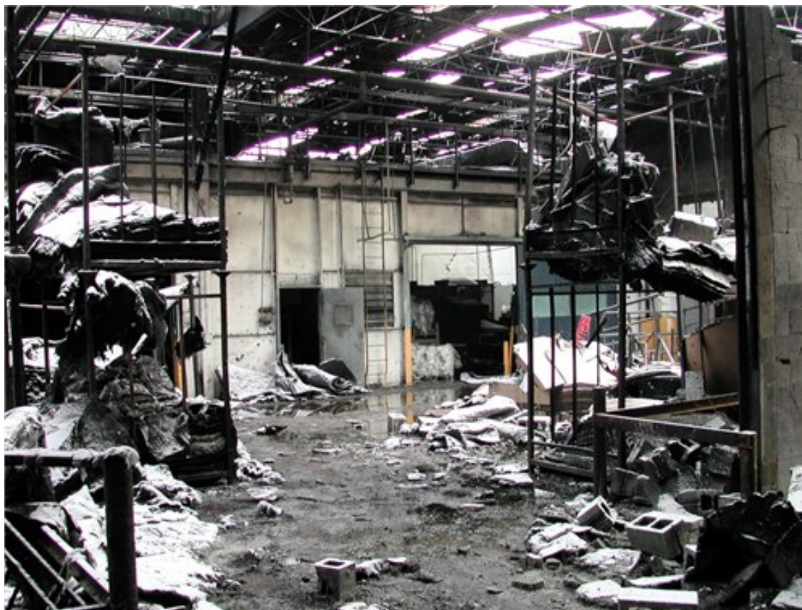
Figure I-2: Results of a dust explosion at CTA Acoustics, Inc., on February 20, 2003. (Source: CSB)
