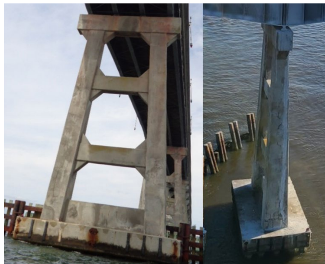
Figure 31 – Concrete deterioration
