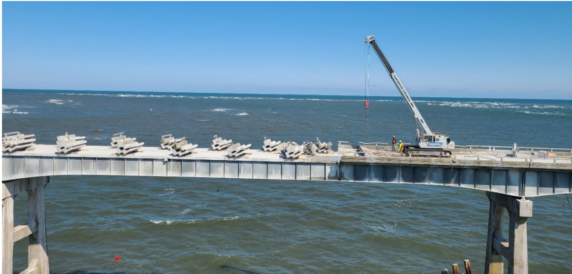
Figure 18 – Demolition of Span 145 (photographed on 3/5/2021 by NCDOT)
