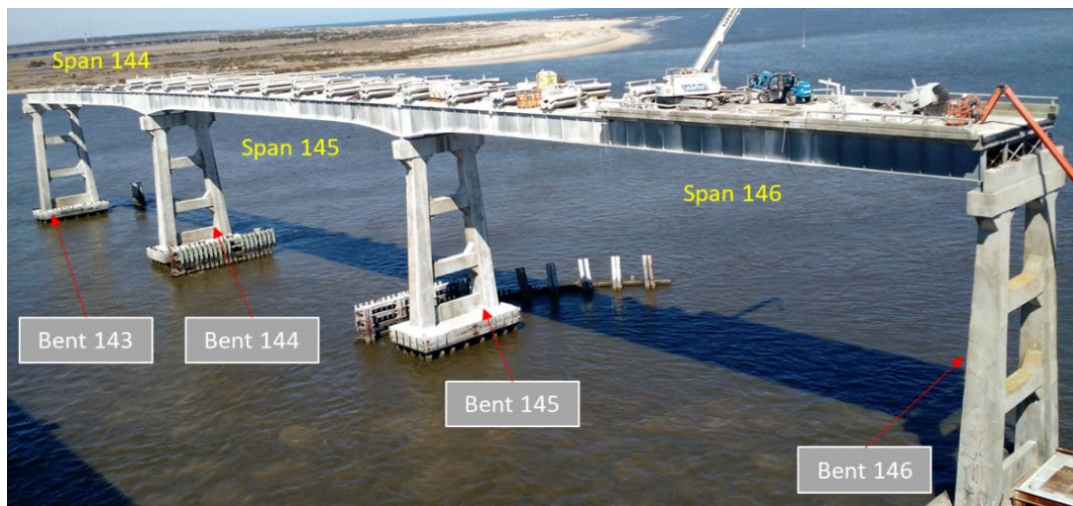
Figure 20 – Three steel girder spans under demolition – Looking north (photographed on 3/11/2021 by NCDOT)
