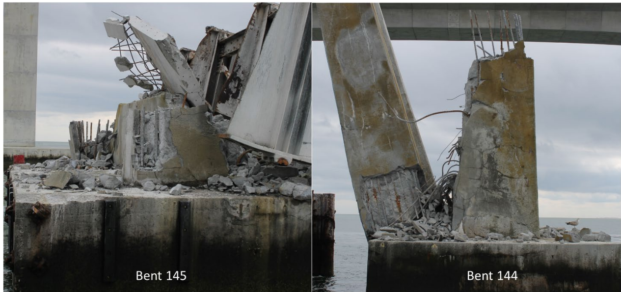
Figure 30 – Collapsed Bent 144/145
