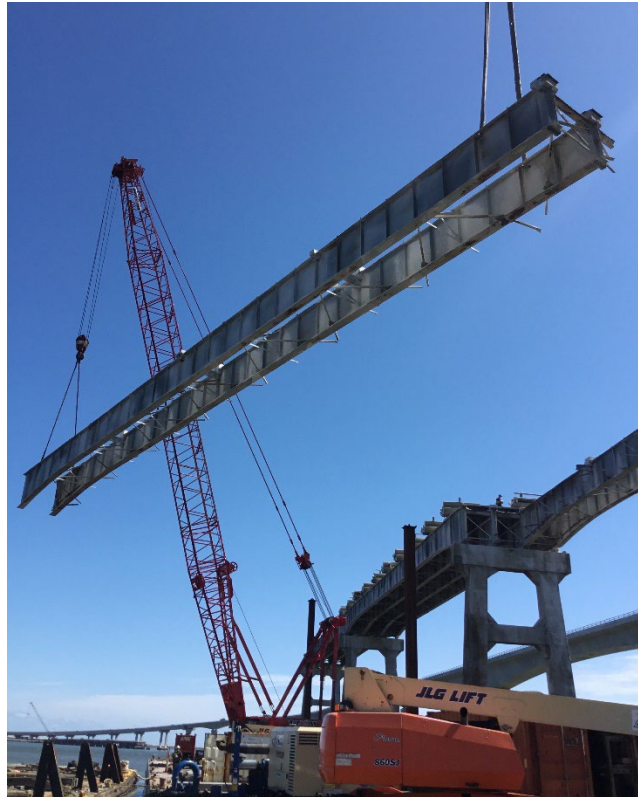
Figure 22 – Removal of Span 144 girders (photographed on 3/30/2021)
