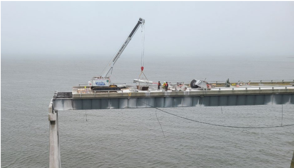
Figure 13 – Demolition of Span 144 (photographed on 2/15/2021 by NCDOT)
