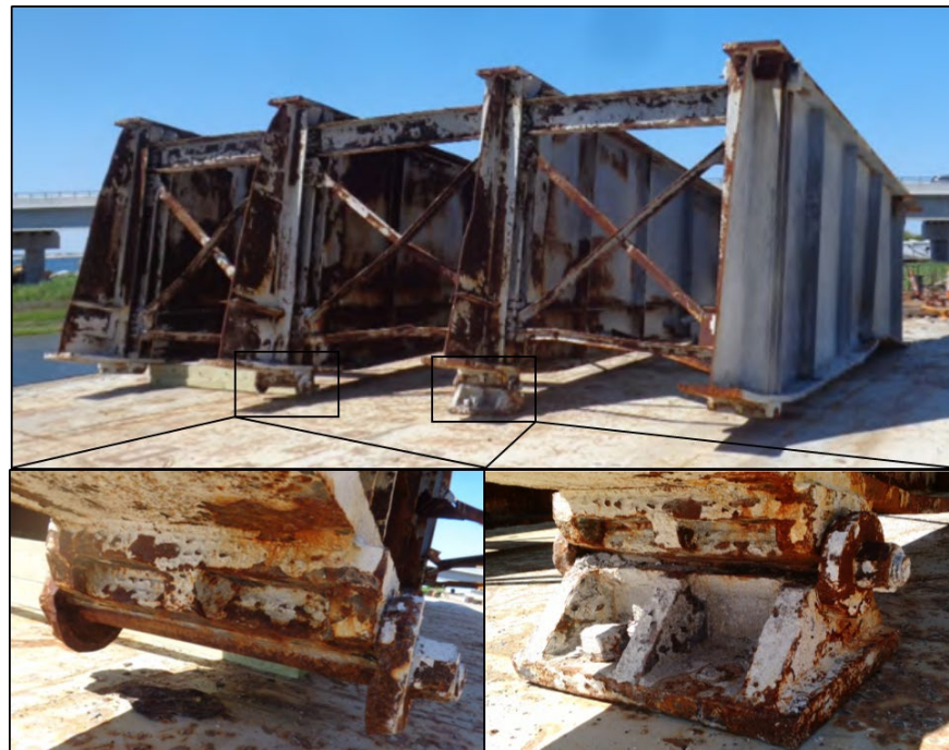
Figure 29 – South girder bearings after the incident
