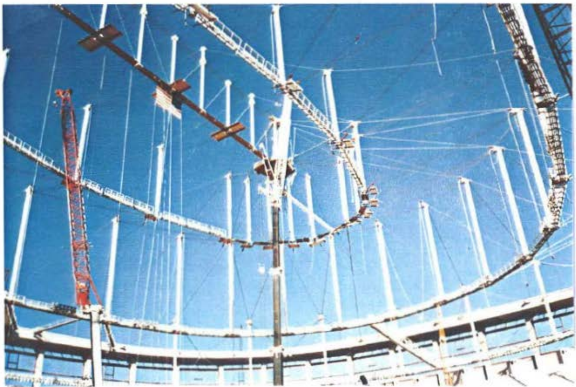
THE COMPLETED ROOF CABLE STRUCTURE AT THE TIME OF THE ACCIDENT. THREE HOOP CABLES, THE POSTS, AND RIDGE CABLES
