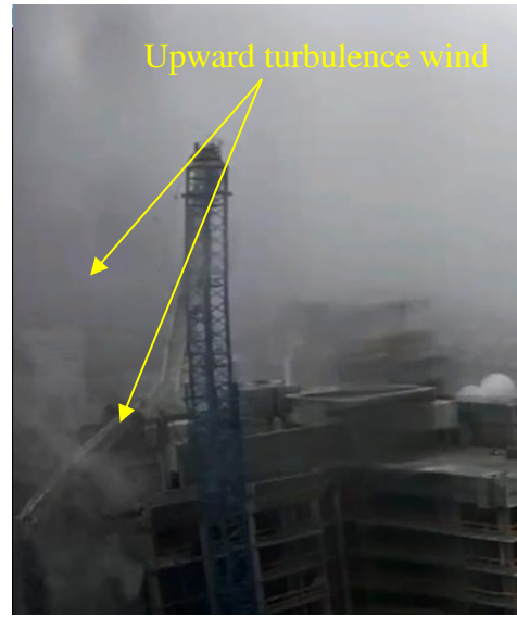
b) Upward turbulence wind detected right after counterweight blocks hit the building
