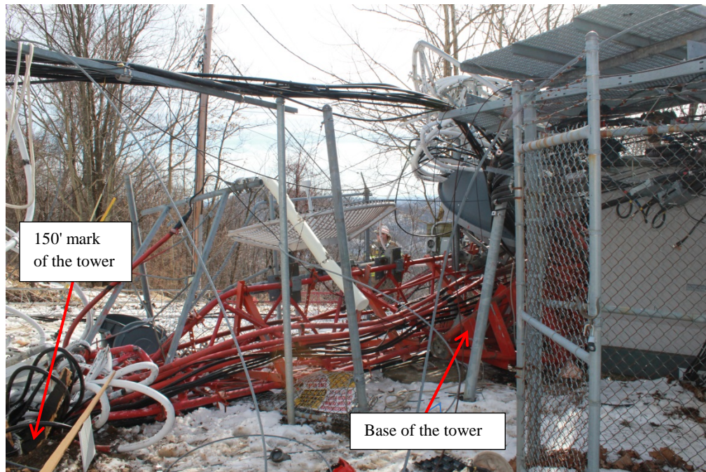
Figure 8. The lower portion of the folded and collapsed tower at its northwest end. Note that the 150' mark of the tower is at the lower-left corner of the photo and the base of the tower is at the lower-middle of the photo (WVSP Photo 5920, looking east).
