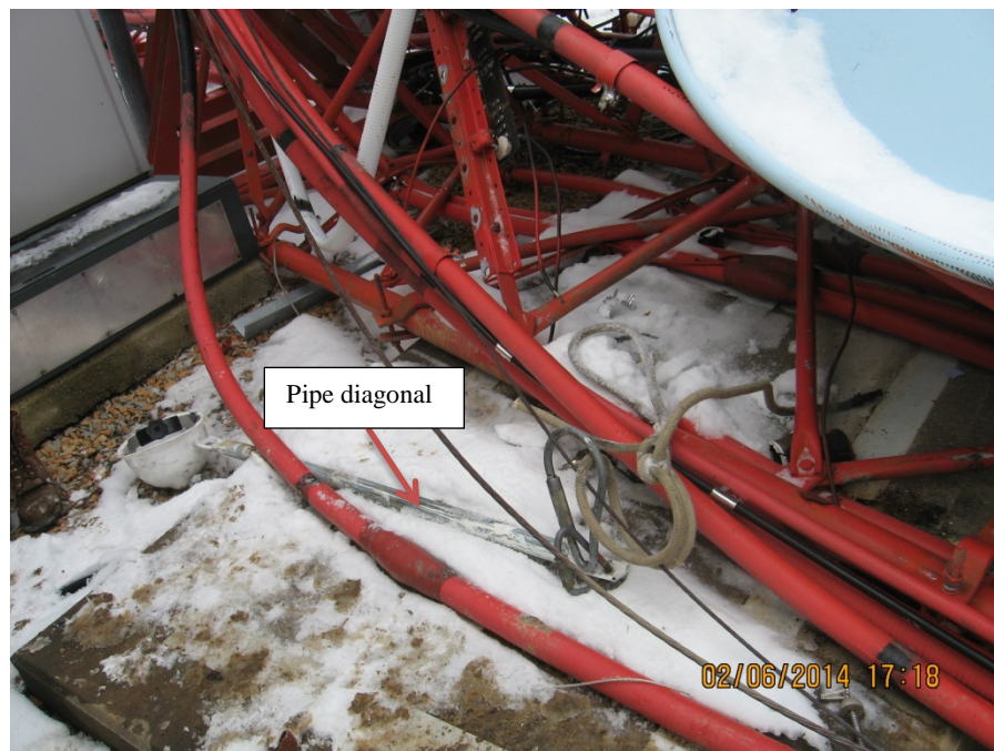
Figure 4. The fifth round diagonal, still fastened to a rope, was found on the way down from the tower.
