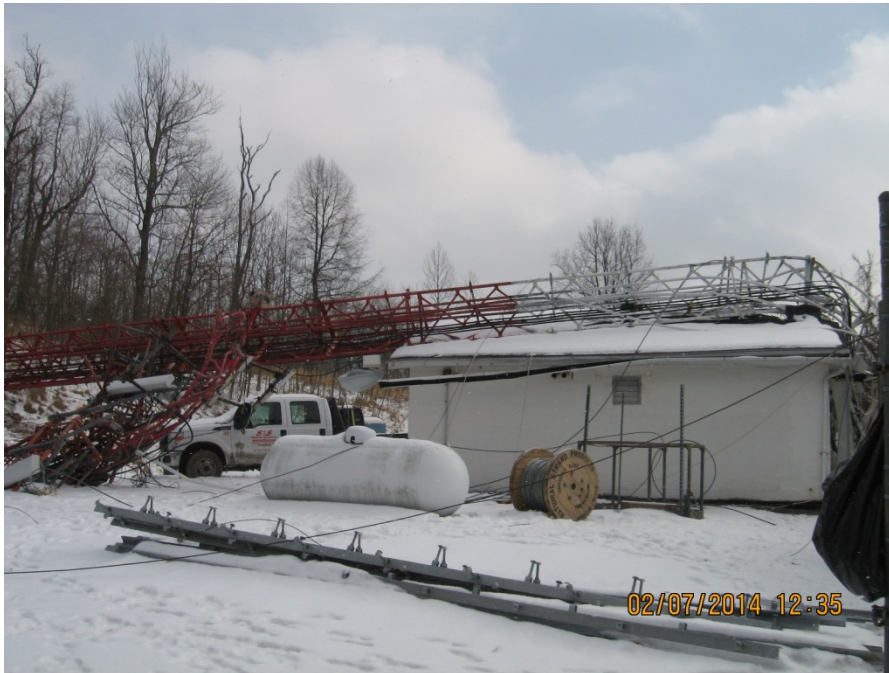
Figure 6. The upper portion of the collapsed tower, approximately from 175' to 240' above the ground (looking northeast).
