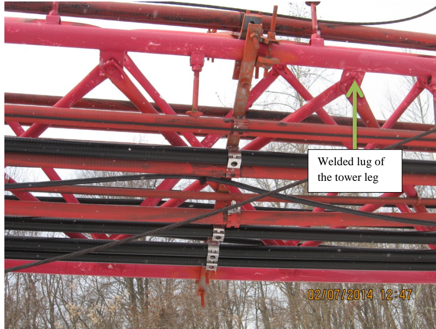
Figure 14. Welded lug of the tower leg; one bolt connects two diagonals.
