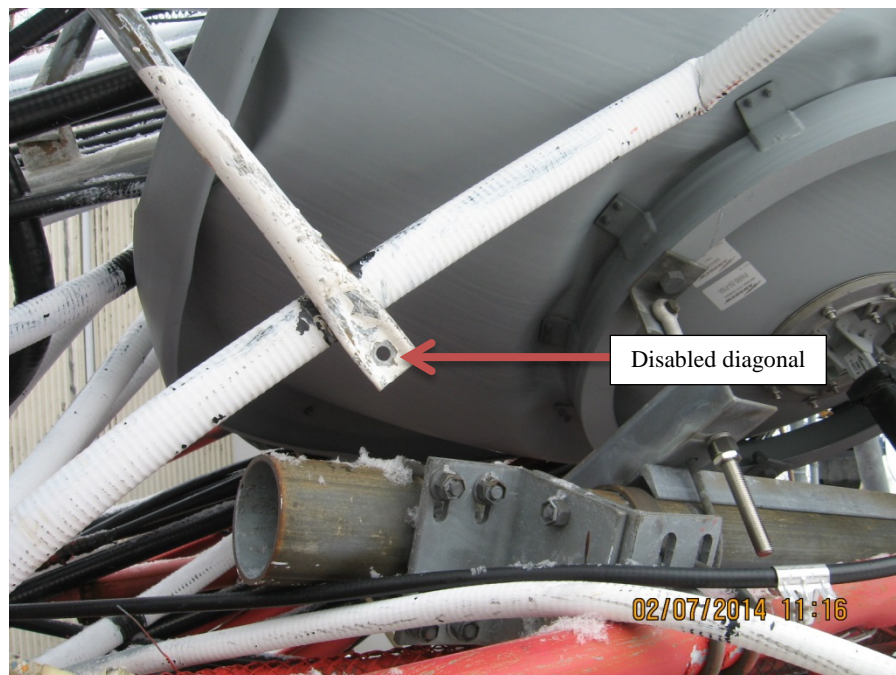
Figure 15. A diagonal disabled by being unbolted from the lug. It is still attached to the tower.
