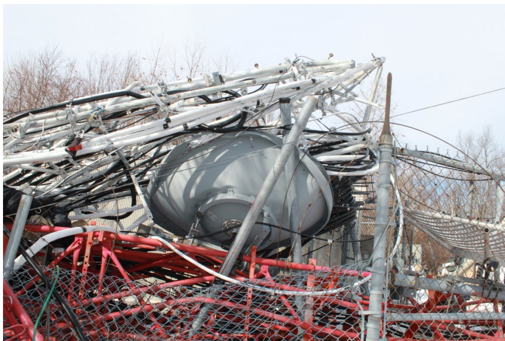
Figure 11. The lower portion of the folded and collapsed tower at the middle of the collapsed pile (WVSP Photo 5868, looking southwest).
