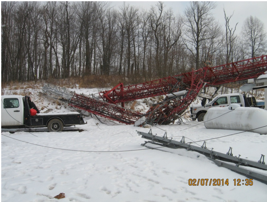
Figure 7. The upper portion of the collapsed tower, approximately from 220' to the top of the tower at 340' above the ground (looking northeast).
