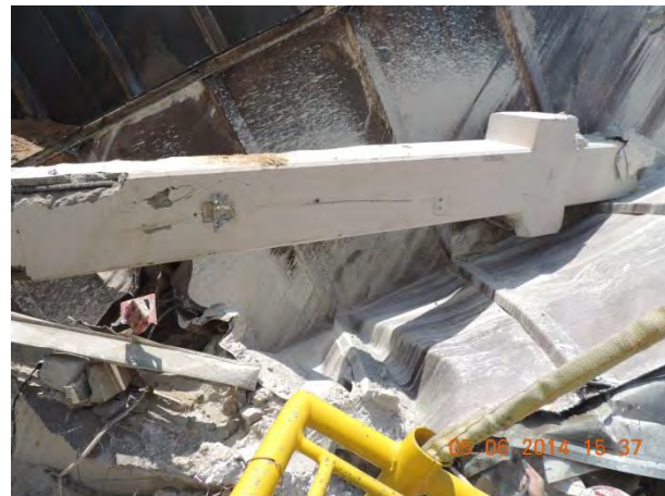
Fig. 99 – NE corner column lying in bin No. 1
