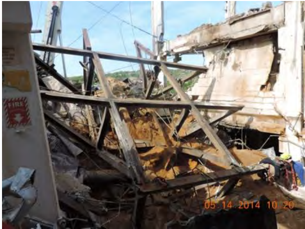
Fig. 104 Interior trusses lying in debris
