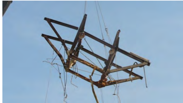
Fig. 105 Interior trusses being retrieved
