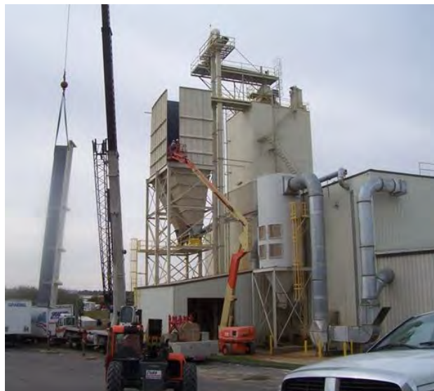
Fig. 7 Two outside bins being added
