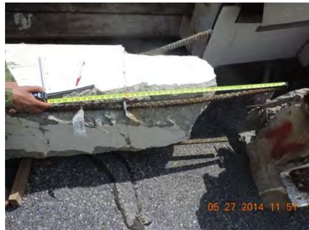
Fig. 103 NE corner column showing inadequate lap splice
