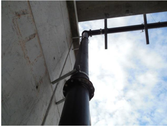
Fig. 15 Water pipe and steel channels support
