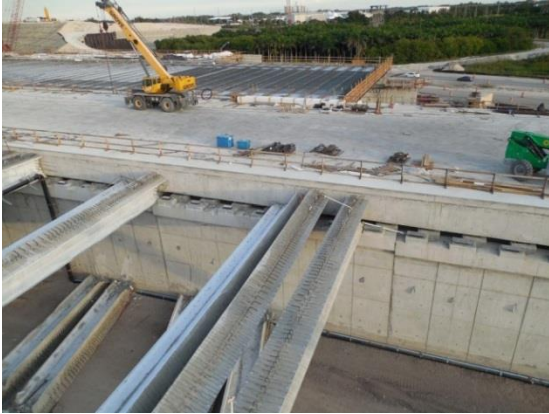
Fig. 11 Displaced beams
