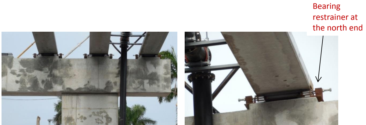
Fig. 30 Pipe support at the north end of cell #2
