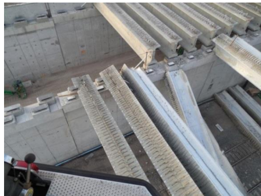
Fig. 8 Fallen and displaced beams
