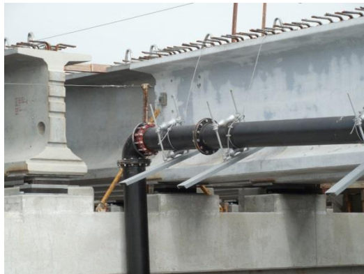
Fig. 14 Water pipe and steel channels support
