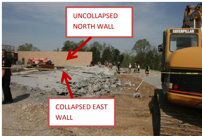
Figure 16 - Collapsed wall
