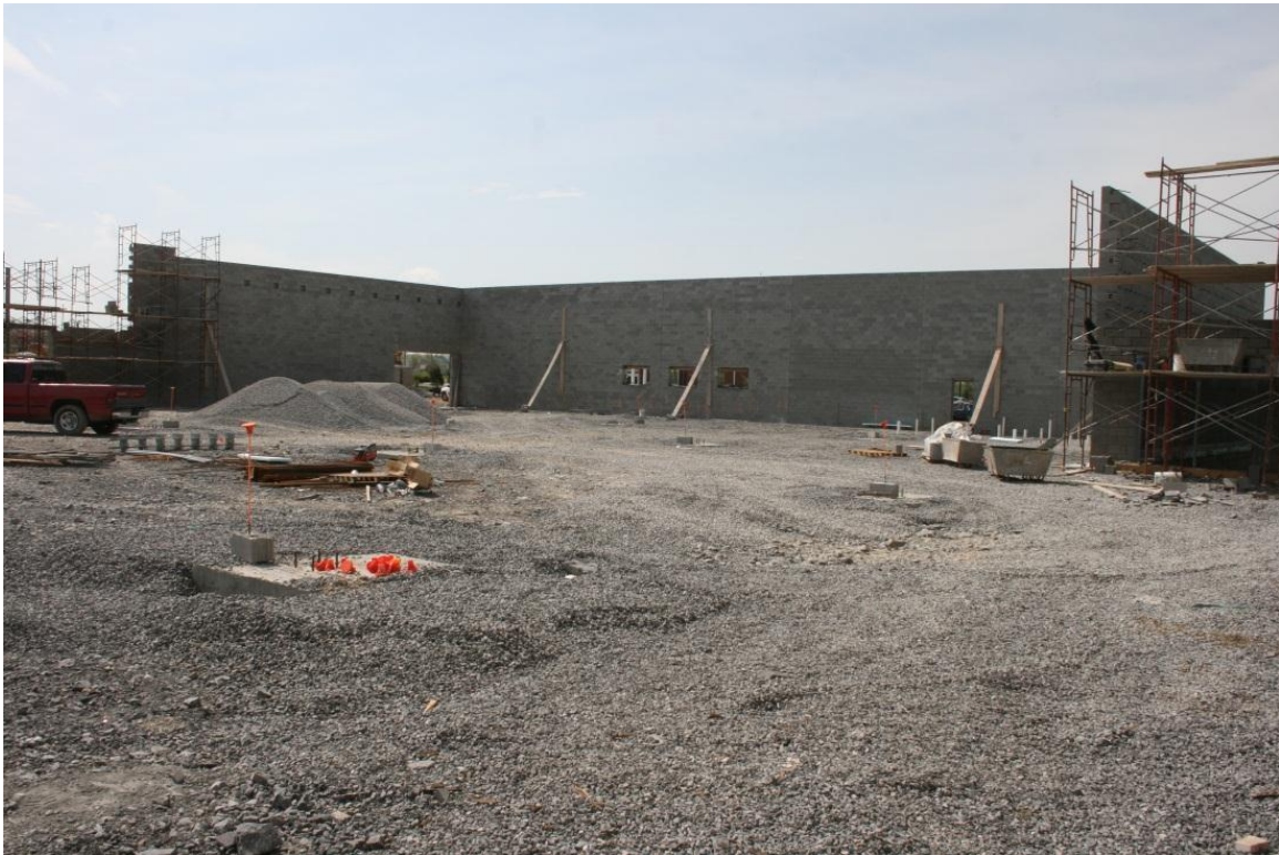
Figure 6 – Typical interior bracing detail
