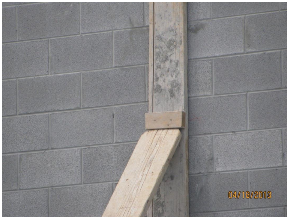
Figure 9 - Top end of brace without positive connection
