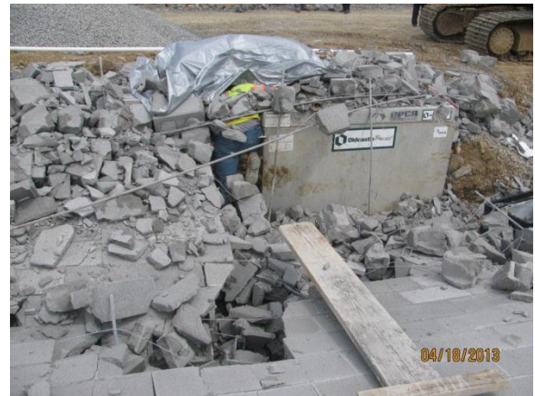
Figure 17 - Collapsed wall
