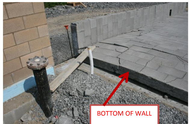
Figure 21 - Collapsed wall
