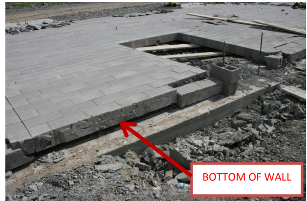
Figure 19 - Collapsed wall
