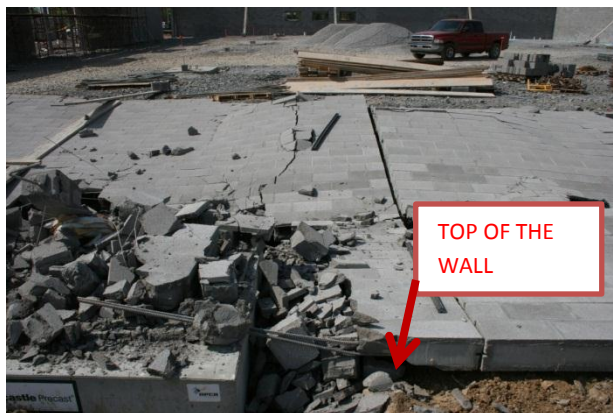
Figure 20 - Collapsed wall
