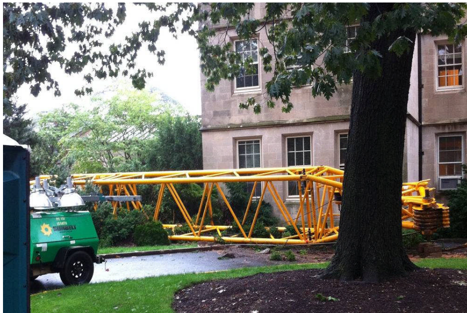
Figure 9. Tip of the Lattice Jib Landed on the Front Yard of the Episcopal Church House (Taken from KCE Structural Engineers, PC).
