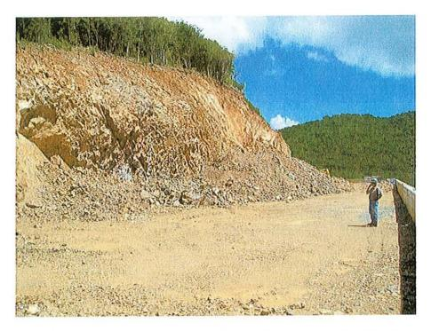
Figure 21. Identifiable Rock Slabs in the Excavation Face South of the Collapsed Area, Looking Toward Northwest.
