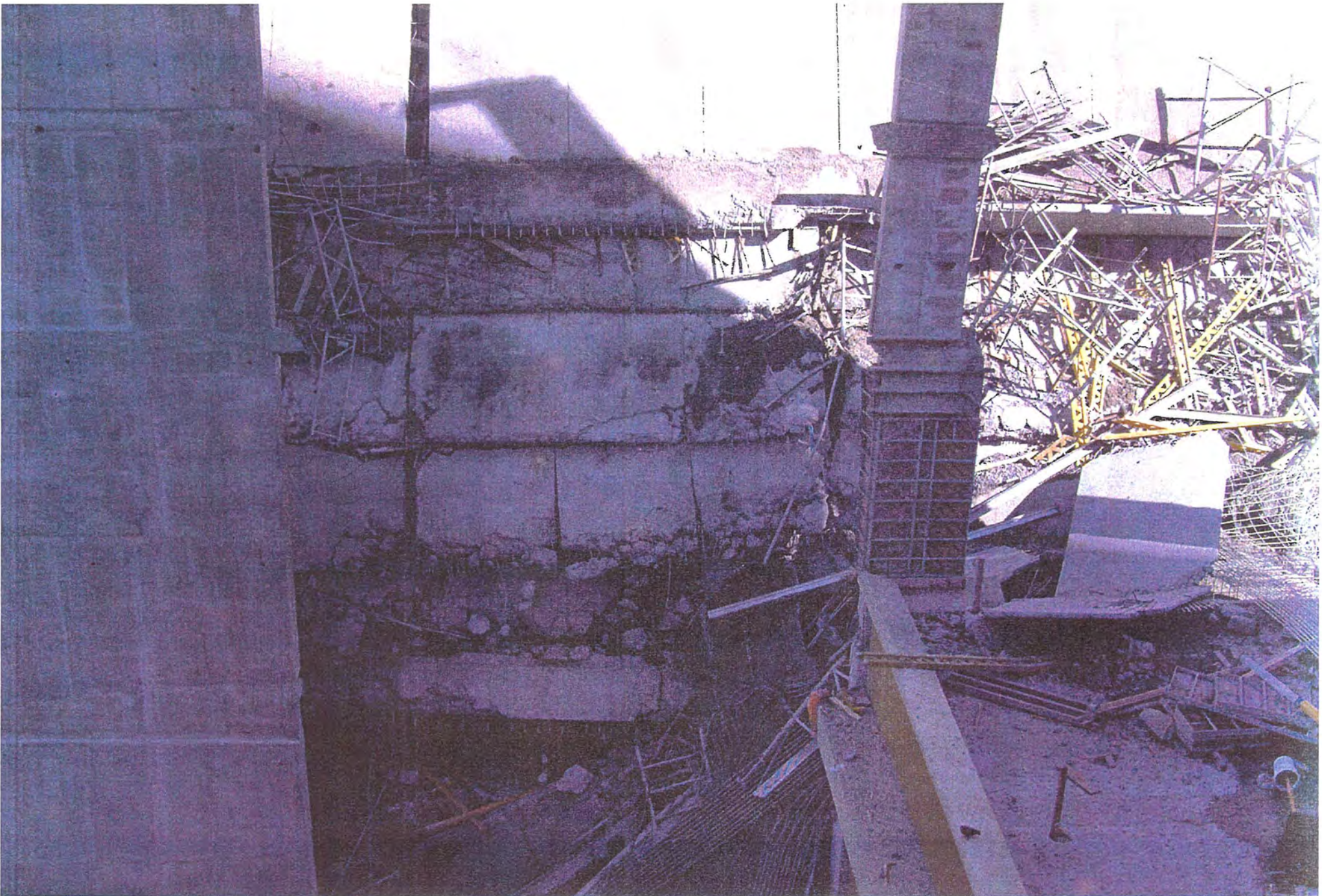
Figure 4. Surface of the Collapse between Shear Wall and Column 1-D (Looking toward Project East).
