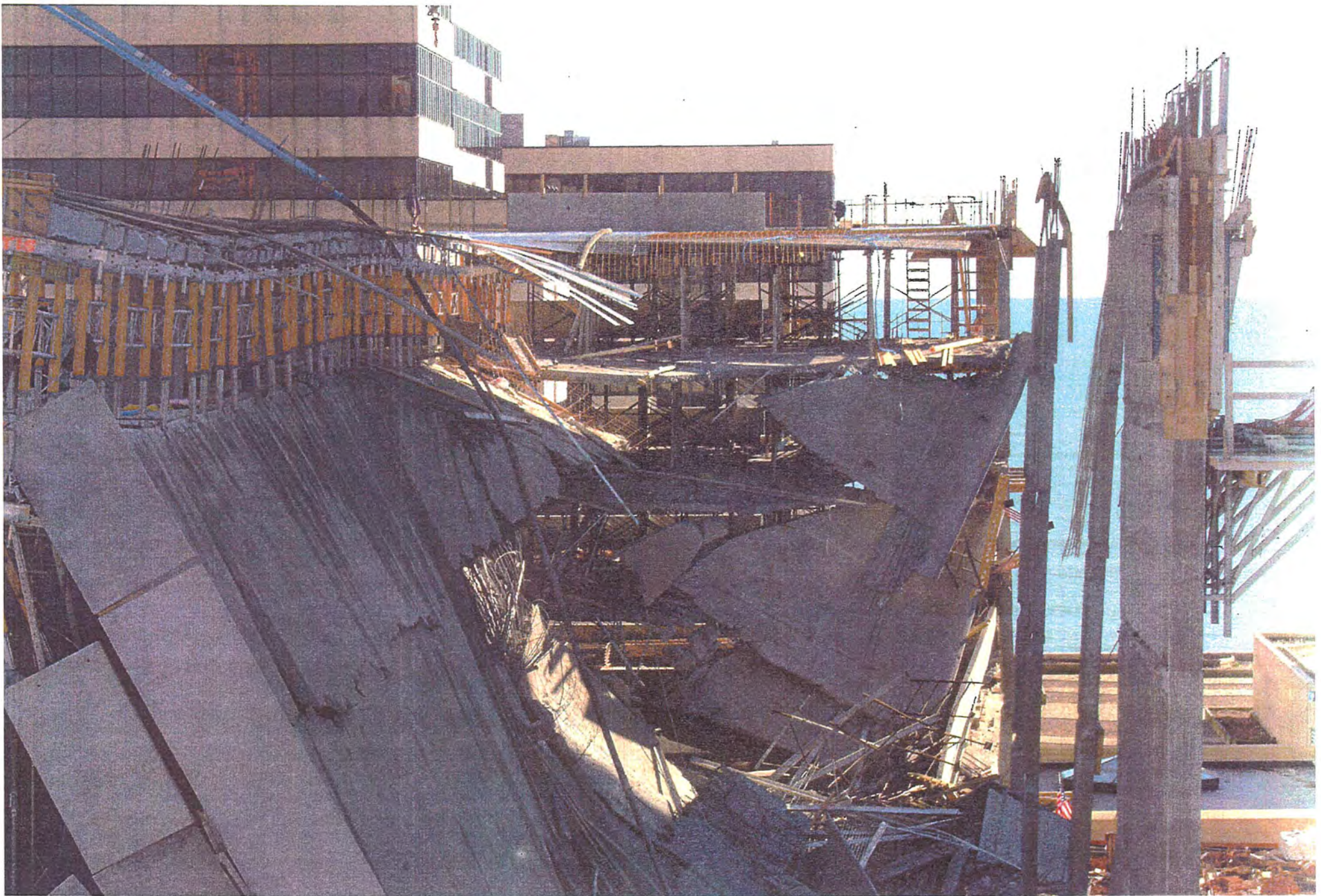
Figure 2. General View of the Collapsed Portion of the Parking Garage (Looking toward the Project Southeast).
